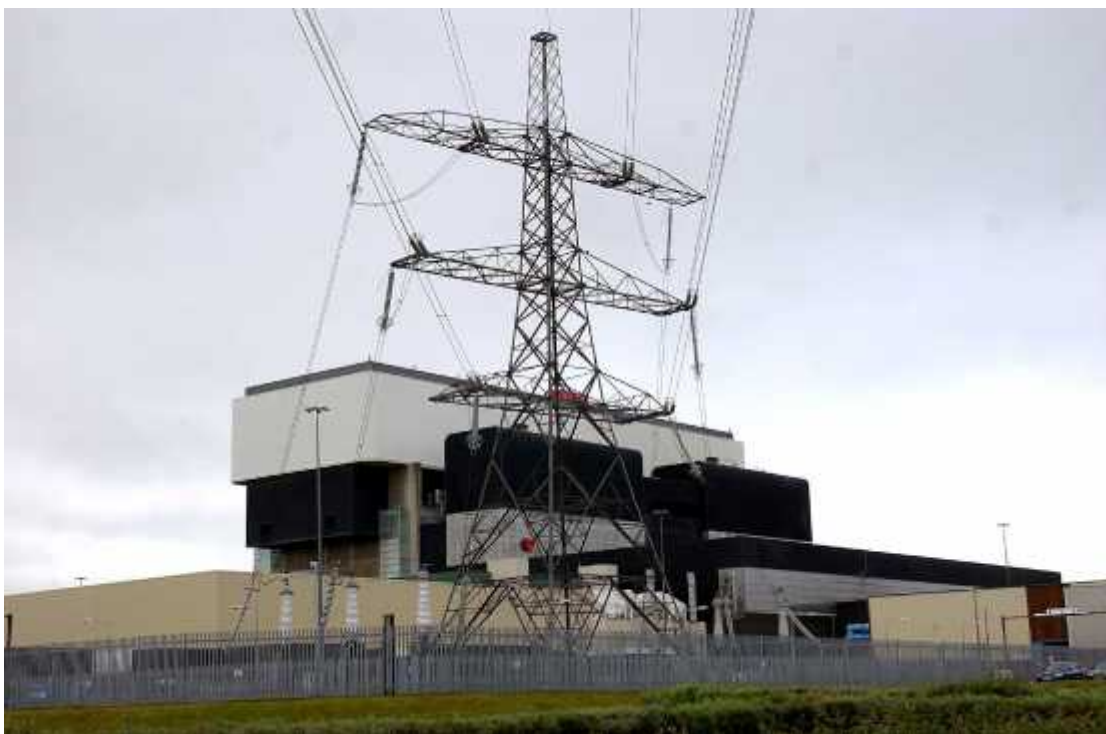
Heysham 2 nuclear power station
